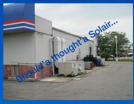
In addition to poor physical appearance this system is vulnerable to coil theft and and vehicles in the parking lot.
